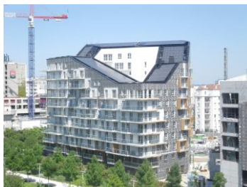
Figure 2 – Low-energy building in Paris' 17 th arrondissement. 96 kW BIPV designed and installed by Sunvie.
